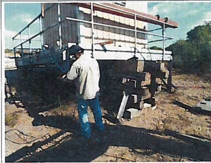
Brieser welder modifying the sampling building supports, looking north
