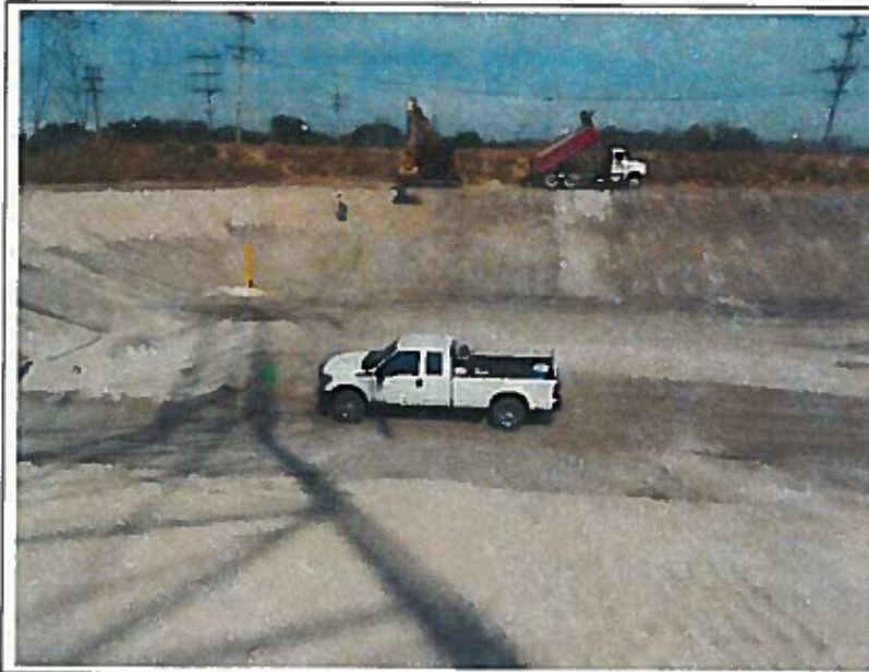
Screening material placement along upper portion of the slope, looking northwest
