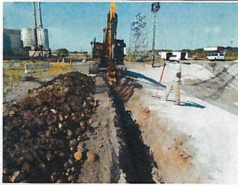
Anchor trench excavation, looking west
