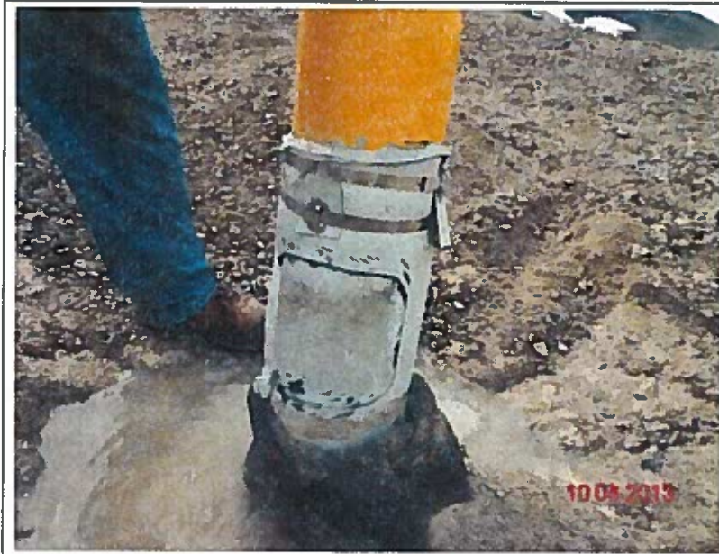
New patch on riser on west slope
