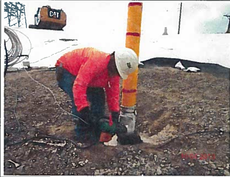
Welding the new patch, looking west
