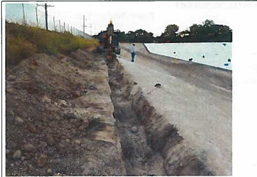
Excavation of the geosynthetics anchor trench, looking northeast
