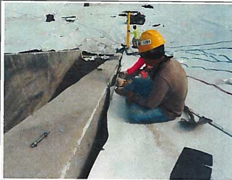
Installation of batten connection to the recycle basin structure, looking east
