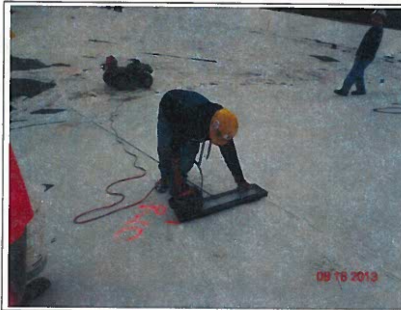
Non-destructive testing geomembrane repairs (vacuum box), looking east
