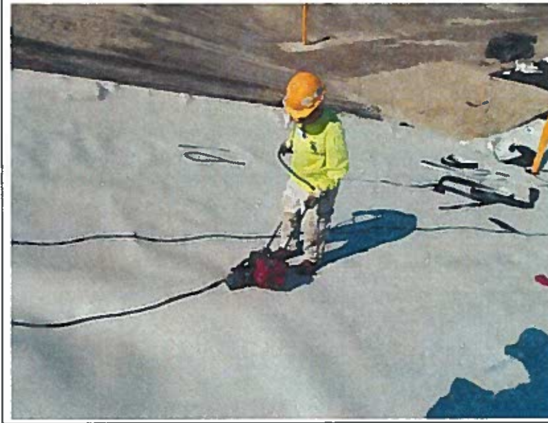
Geomembrane production seaming, looking north
