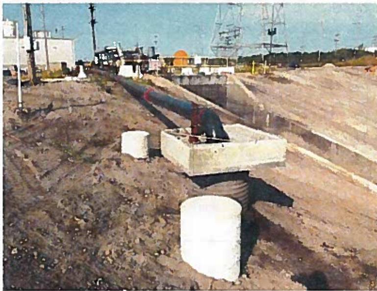
View of Sampling Building downslope cylindrical foundations, facing west
