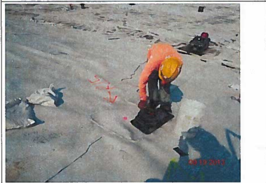
Vacuum testing along southwest slope
