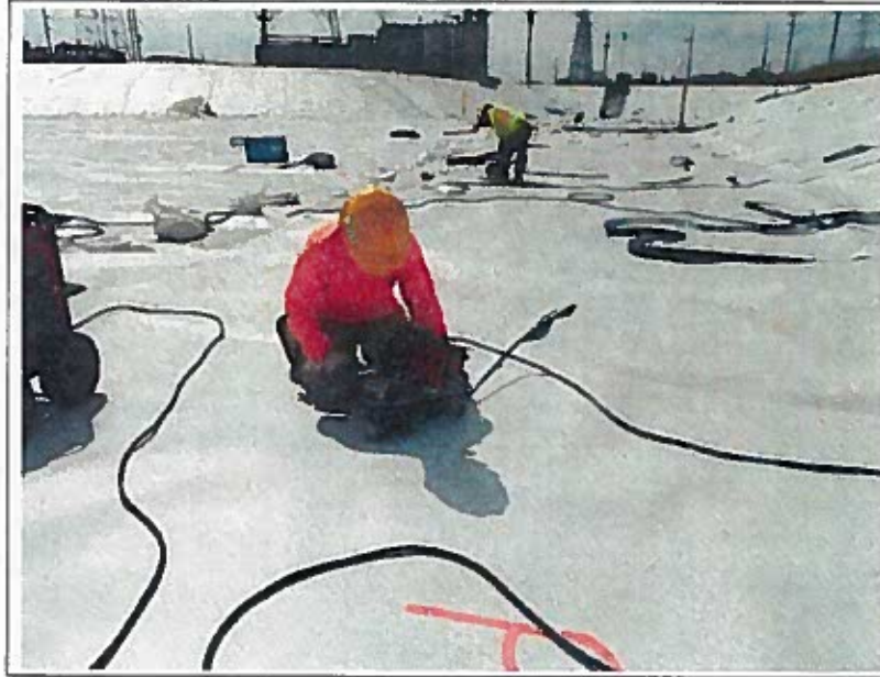
Geomembrane trial weld prior to production seaming, looking southwest
