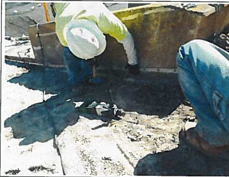
Preparation of batten strip connection to the inlet structure, looking south
