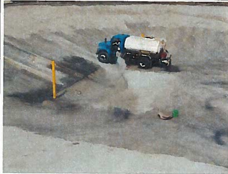
Moisture conditioning screenings placed in sump prior to compaction, looking northwest
