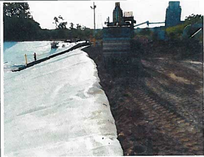
Backfilling anchor trench, looking south
