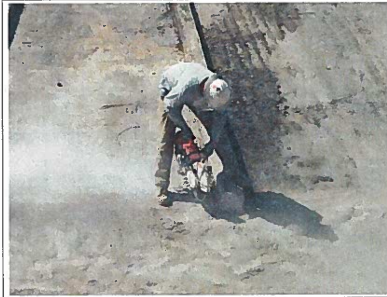
Preparation of concrete surface for geomembrane batten connection, looking west
