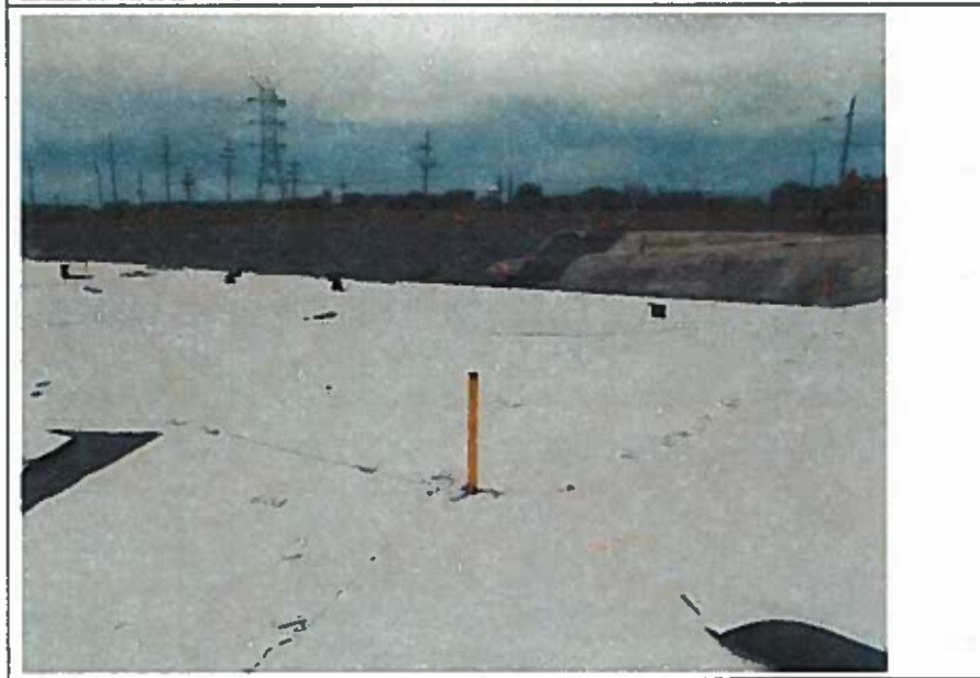
Installation of geotextile over the remaining pond area, looking northwest
