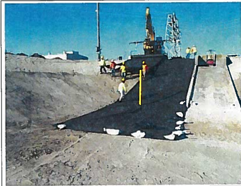
Geotextile deployment, looking southwest
