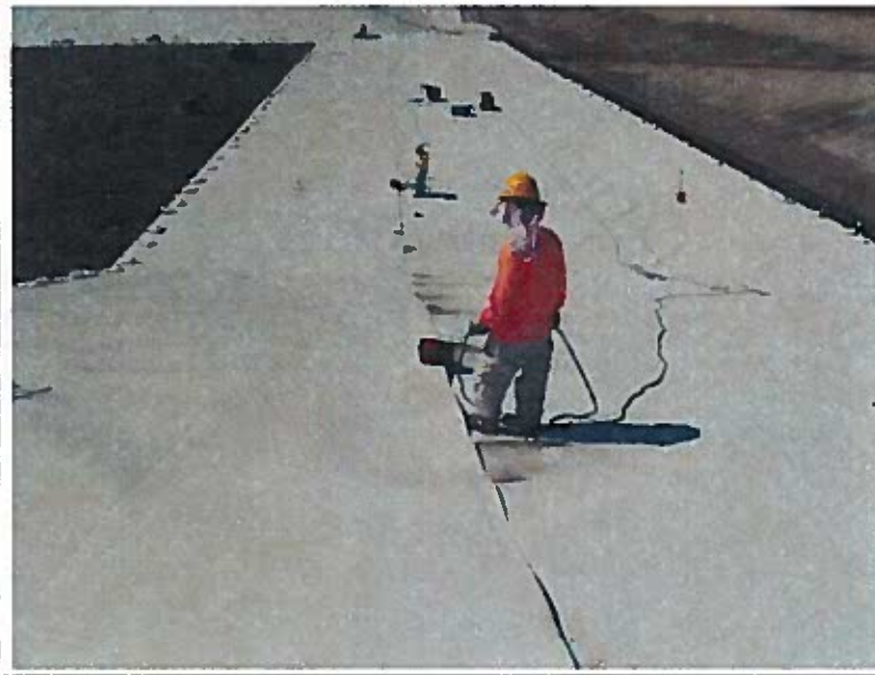
Panel seaming, looking west
