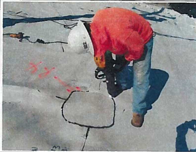
Extrusion welding geomembrane repair, looking east
