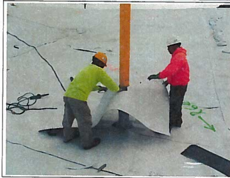
Installing geomembrane pipe boot around marker post, looking east
