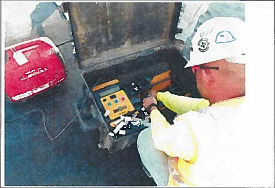
Testing trial welds in the tensiometer, looking southeast
