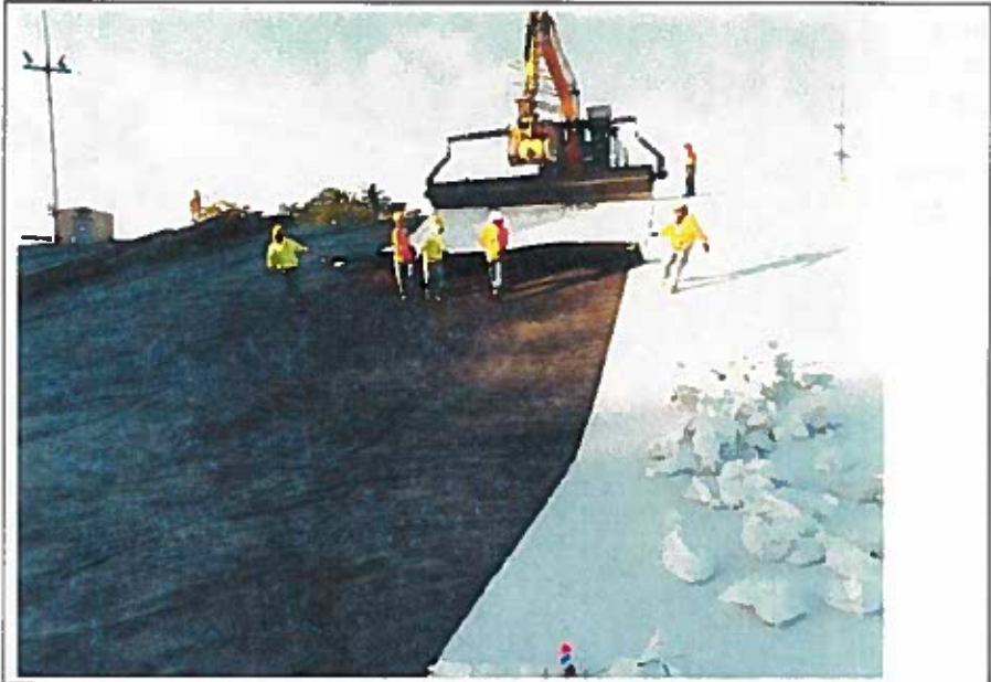
Geomembrane panel deployment, looking southwest
