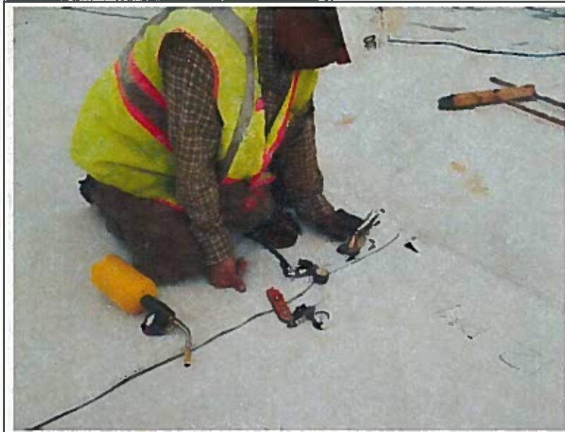
Non-destructive testing geomembrane fusion welded seam, looking southeast
