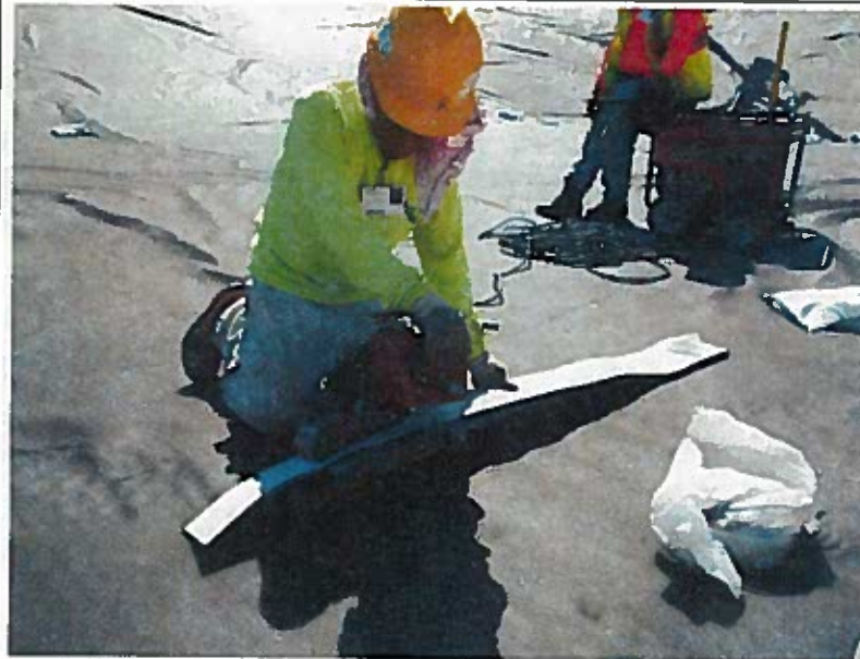
Preparing geomembrane trial weld, looking north
