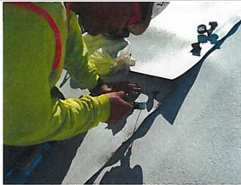
Performing non-destructive air testing of the geomembrane fusion welded seams
